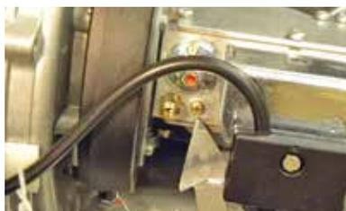
Gas:Air ratio adjustment screw
