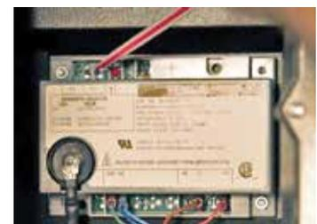
Fenwal ignition module - Microamp ( $\mu\text{A}$ ) test points are shown at top left corner of module (beside red L.E.D.)
