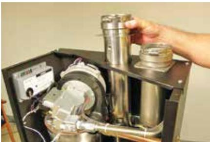
*Removing vent stack*
