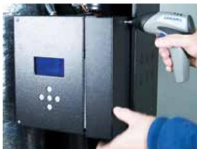
Removing wiring box covers
