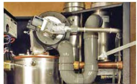
*Combustion air intake riser*
