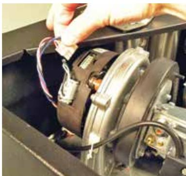
Unplugging fan control harness plug will drive the fan into manual high speed operation for vent leak test
