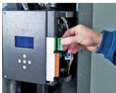
Line voltage load pump terminals
