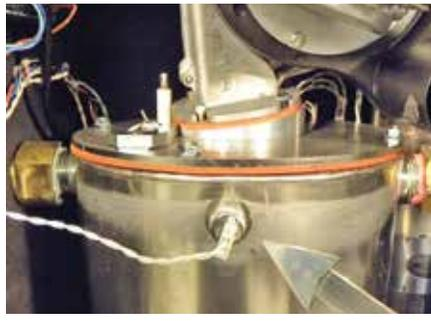
*Outlet (supply) water temperature sensor*
