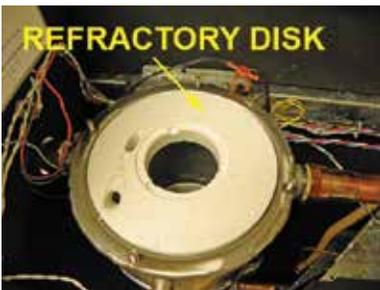
Combustion Chamber Refractory
