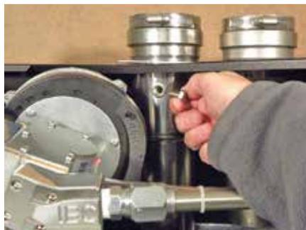
*Removing vent stack test port plug*
