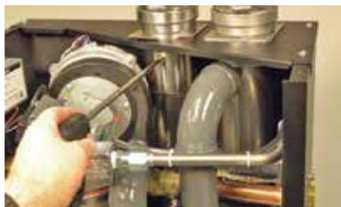
Flue gas test port plug
