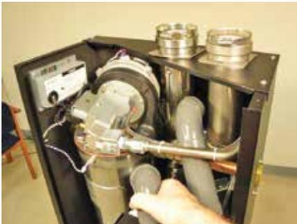
*Removing combustion air intake riser*
