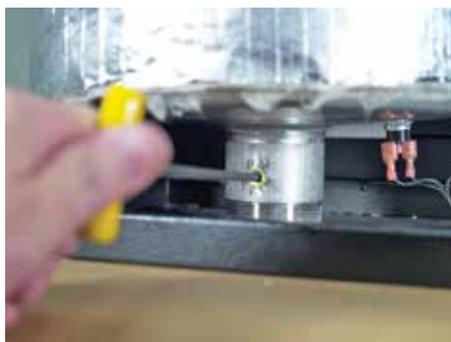
Removal of flue gas test port plug
