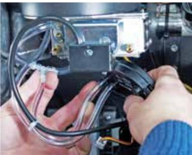
Air pressure sensor removal showing reference line connections
