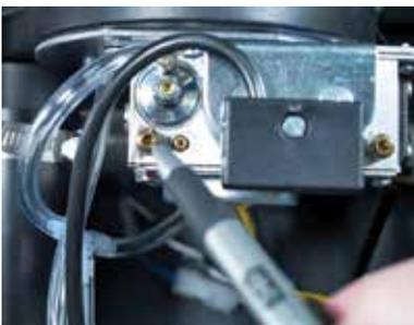
Manifold pressure test port
