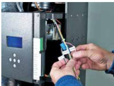
Line voltage leads for power supply, primary pump and variable speed output
