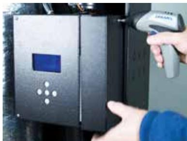
Removing wiring box cover
