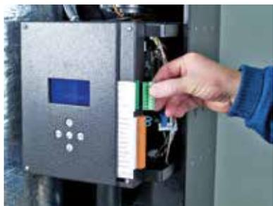
Line voltage load pump terminal strip
