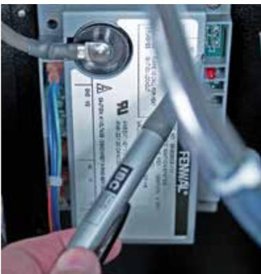
Fenwal ignition module - Microamp ( $\mu A$ ) test points are shown at top right corner of module (above red L.E.D.)
