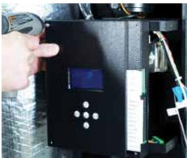
Removing circuit board cover
