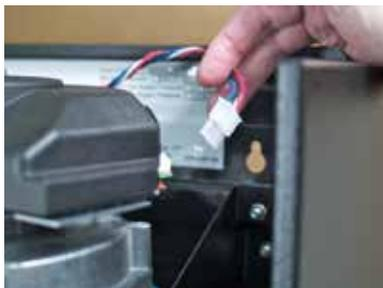
Unplugging fan control harness plug will drive the fan into manual high speed operation for vent leak test
