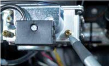
Inlet gas supply pressure test port
