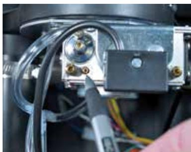
Gas:Air ratio adjustment screw
